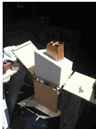
13. cast ready // curing time : 1 day
