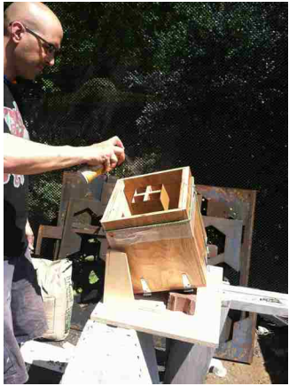
6. applying release agent : PAM
